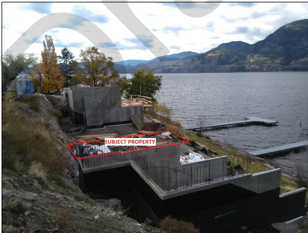
Figure 5: North View of Subject Property
